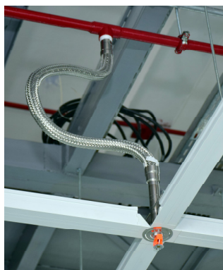
Typ. Clean Room sprinkler installation
